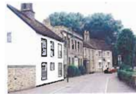
Brook Street Heritage
